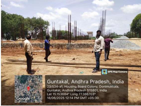
Hostel Construction Work
