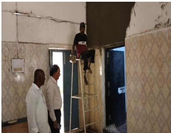
Women's Waiting Hall Renovation Work
